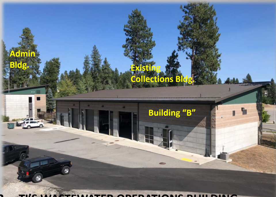
PHASE 2 – TI'S WASTEWATER OPERATIONS BUILDING
